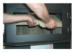
Important: push both baffle bricks so they are tight against the side walls.
